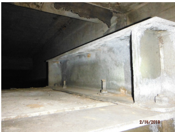
Photo 5. LBP Positive Large Repair Beam
