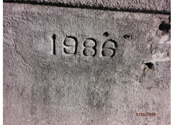
Photo 2. Date Stamp on Bridge
