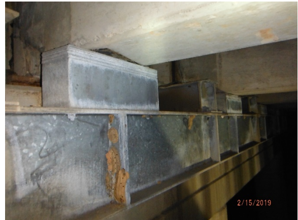
Photo 4. LBP Positive Small Repair Beam
