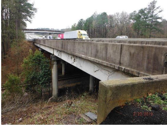
Photo 1. East Side View of Bridge
